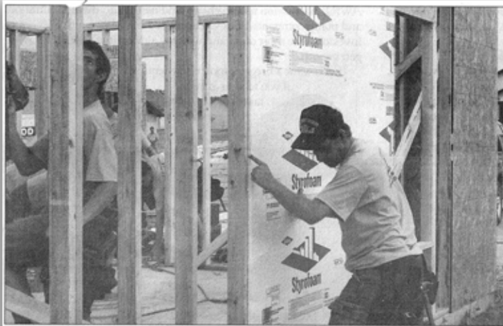
Southcreek Construction's framing crew working on a Habitat for Humanity home.
